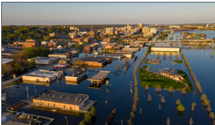
Figure 15 | 2019 flood looking East over Downtown Davenport and River Drive
